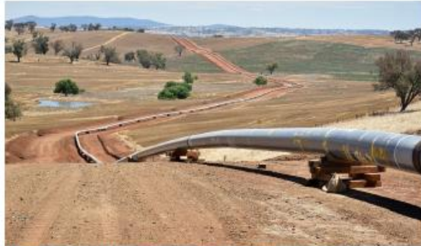
Pipeline under construction, prior to being lowered into the ground.
